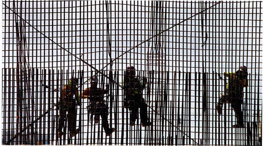
Construction workers are seen as they work with steel rebar during the construction of a building on May 17, 2019, in Miami, Florida. The Trump administration had just announced that it would be lifting tariffs on Canadian and Mexican steel imports, nearly a year after imposing the duties. (JOE RAEDLE/GETTY IMAGES)
